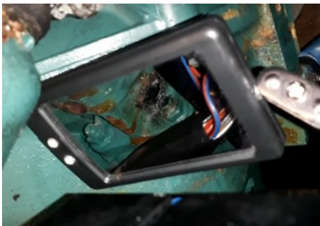
Hole in exhaust elbow
